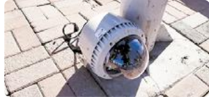
Structural damage of the equipment by vibrations
